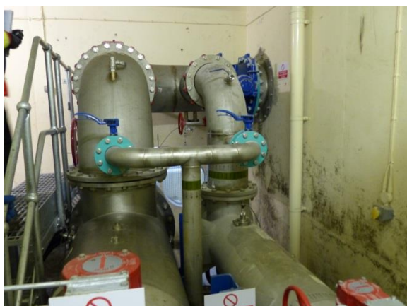
Tullich UV Treatment Unit
