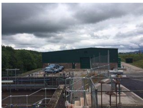
Killylour WTW – completed May 2016
