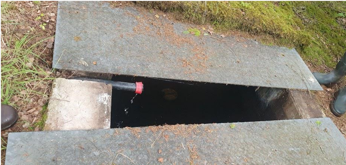
Figure 12: A Poorly Sealed Collecting Chamber
