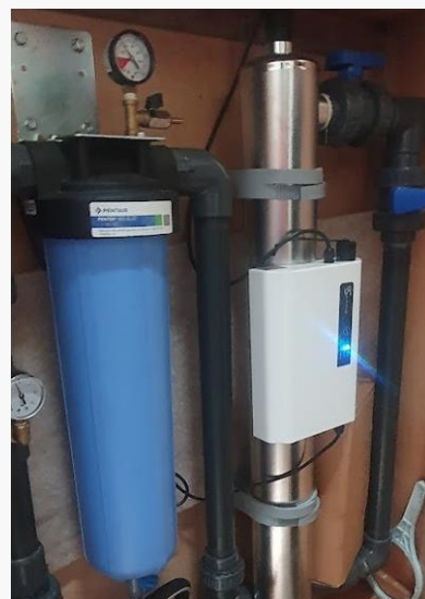
Figure 14: UV treatment to remove bacterial contamination
