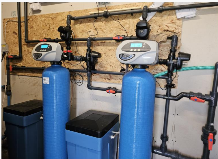
Figure 13: Ion exchange filters to remove manganese and iron
