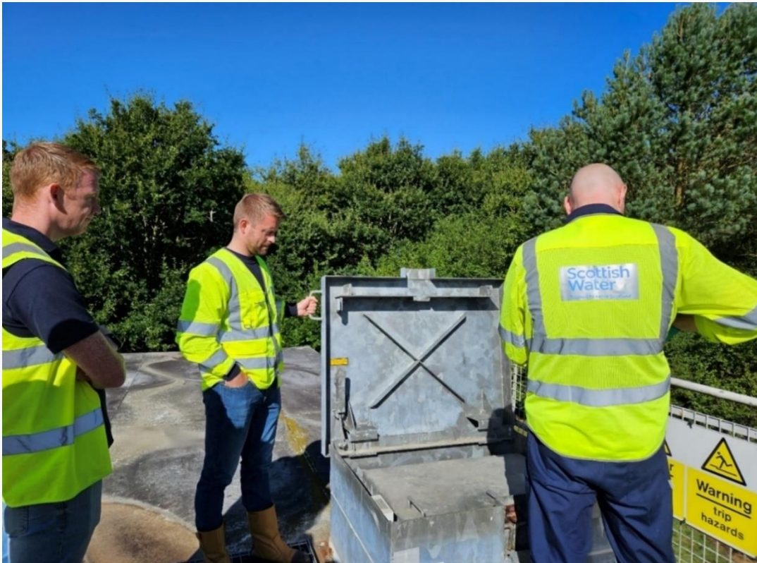
Figure 5 Scottish Water staff inspecting a service reservoir hatch.
