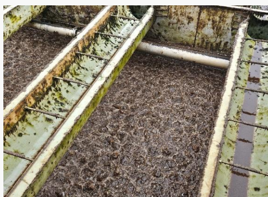
Figure 9 A filter backwash at a WTW.
