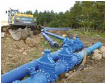
47,000km Water Mains
