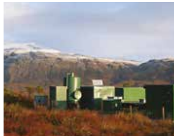
242 Water Treatment Works
