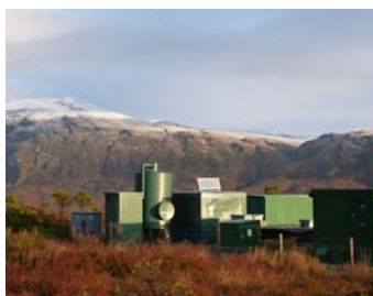
267 Water Treatment Works
