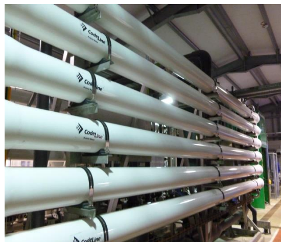
Balmichael WTW membrane treatment units
