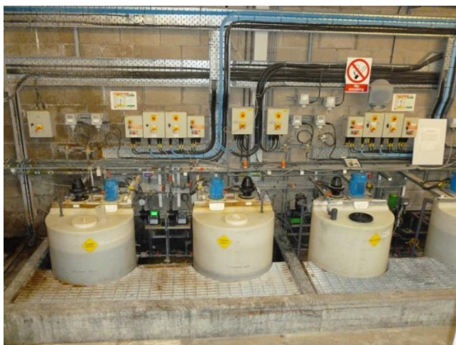
Chemical dosing equipment
