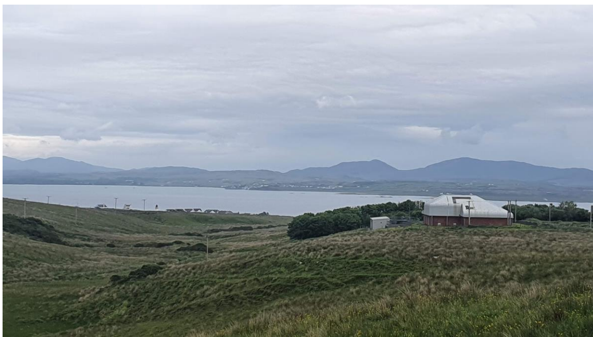
Image 9 Water Treatment Works on Islay
