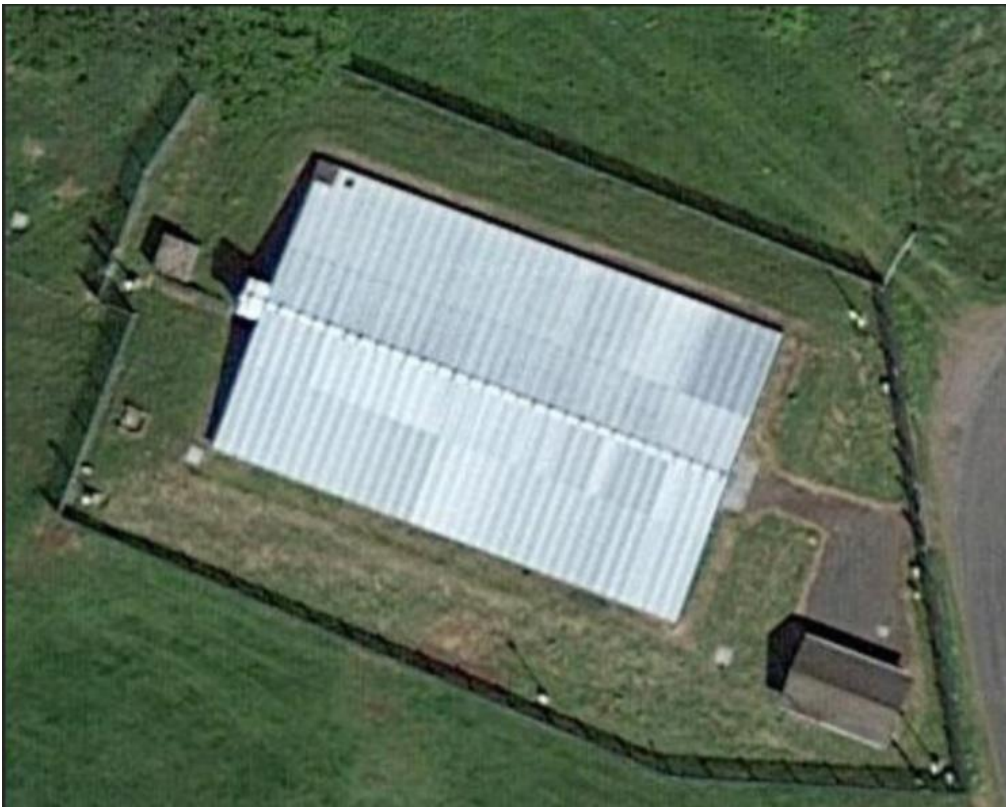
Image 7 Aerial view of Darvel SR (Repaired) – Image supplied by Scottish Water
