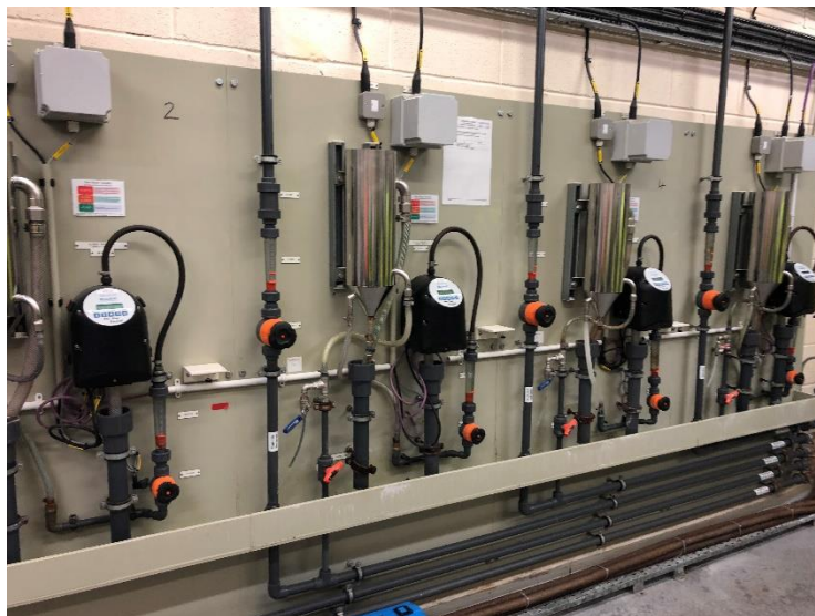
Image 17 Borehole turbidity monitors
