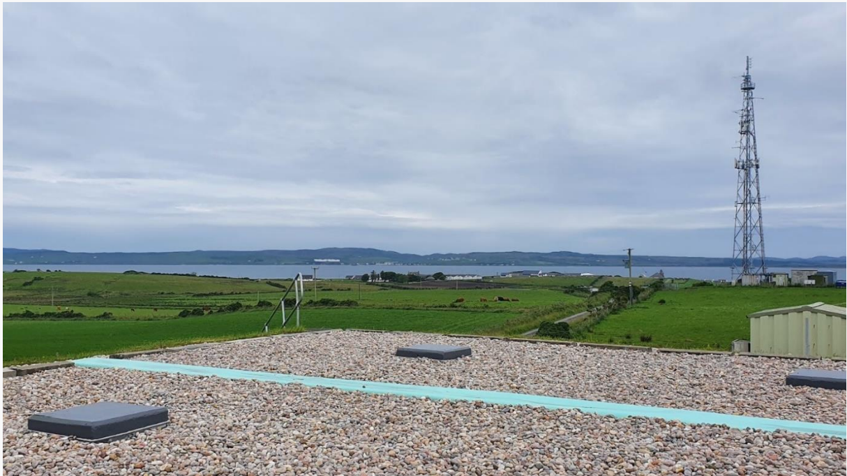
Figure 4 View from the top of a SR.
