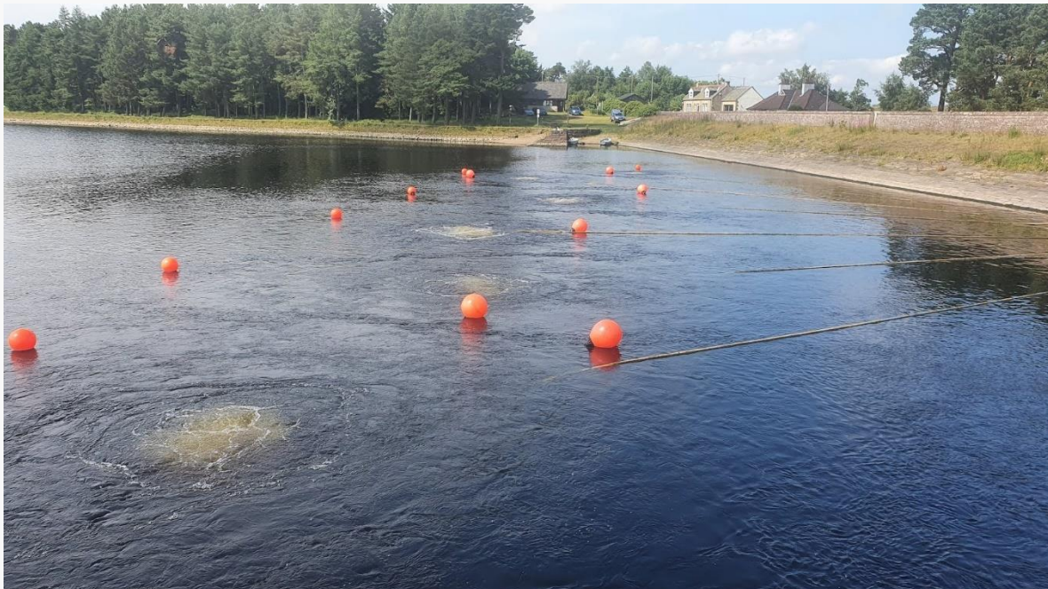
Figure 8 Bubble curtain used to disrupt algal growth.
