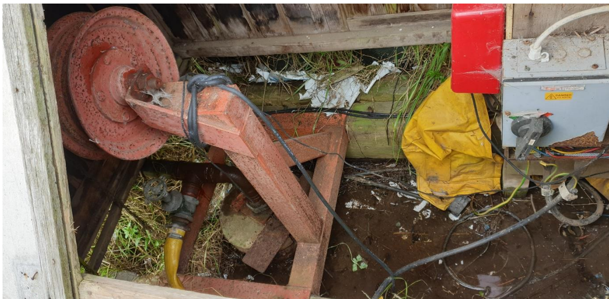
Figure 15: Borehole headworks
