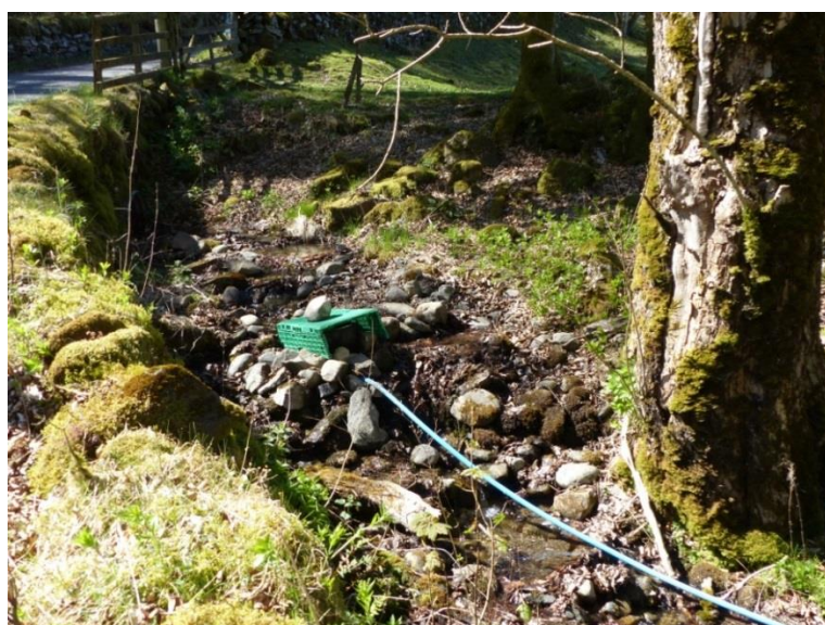
A rudimentary, and vulnerable, surface water abstraction point for a small private water supply
