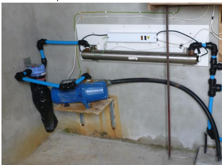
Simple UV Disinfection process at an island PWS
