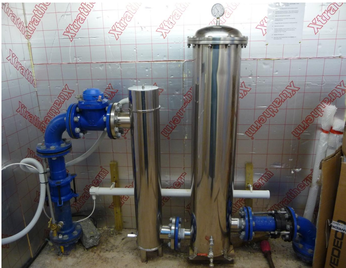
Simple, but well installed and managed Type A PWS
