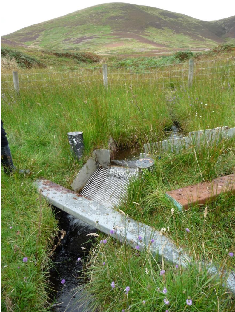
PWS intake in upland area, showing screen to filter debris
