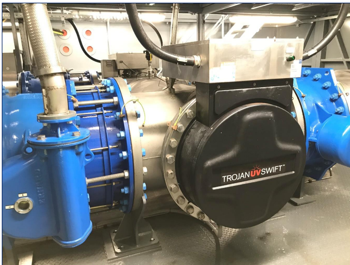
Image 2 UV filters like this one inactivate Cryptosporidium oocysts which may be present in source waters.
