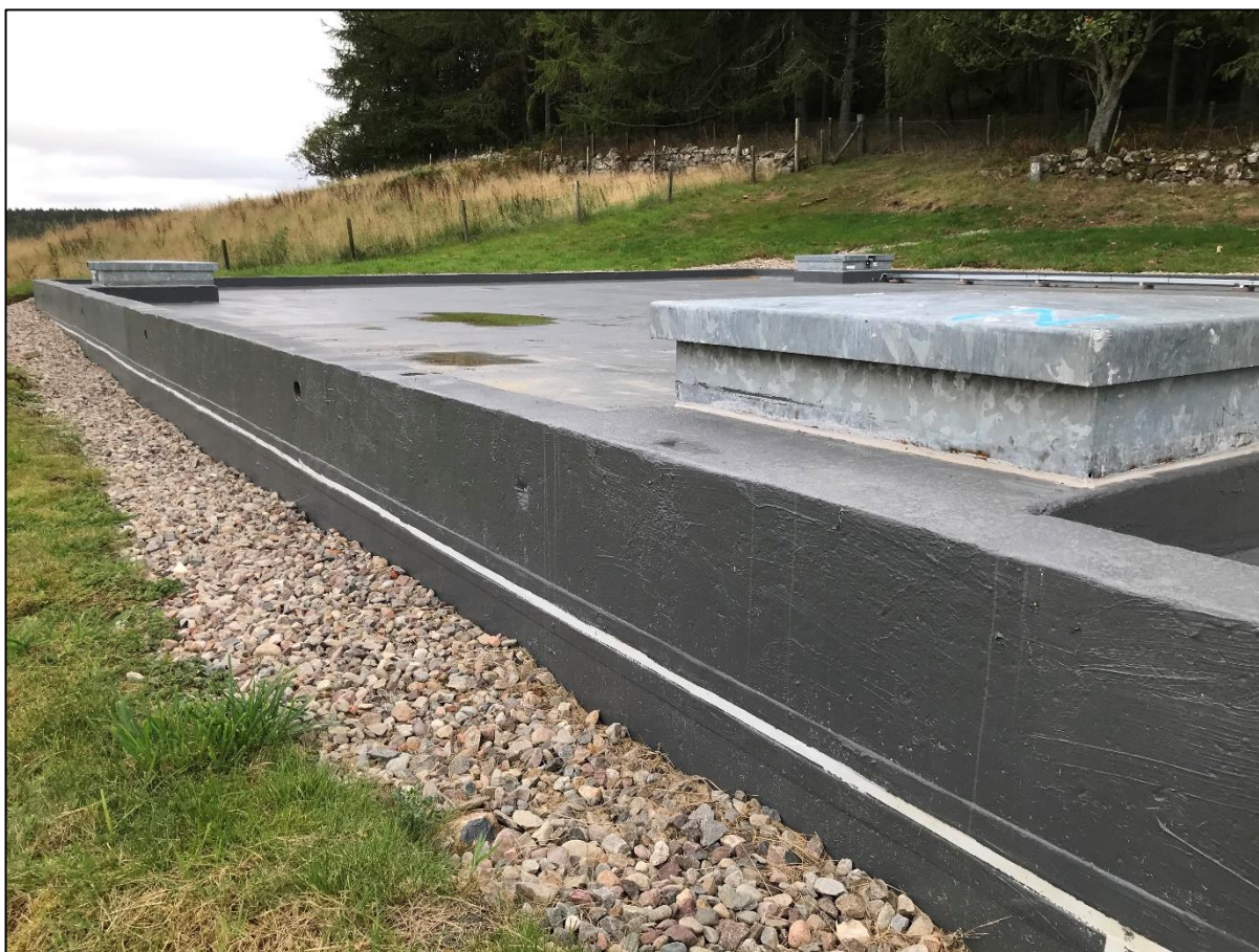
Image 4 Recently refurbished Torphins Cockardie SR, showing renewed joint seals, surface coating and peripheral drainage to prevent ingress of surface water. Service Reservoirs need to be maintained regularly to reduce risk of contamination.
