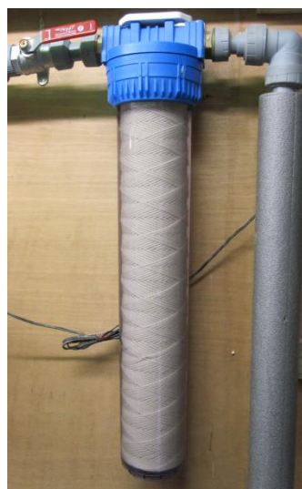
Example of a wound fibre cartridge filter in newly replaced condition in its housing.
