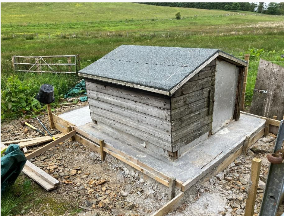
Figure 22 An example of mitigation (housing) to protect a private water supply source.
