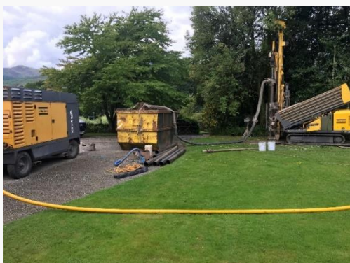
Figure 1 Drilling a new borehole.
