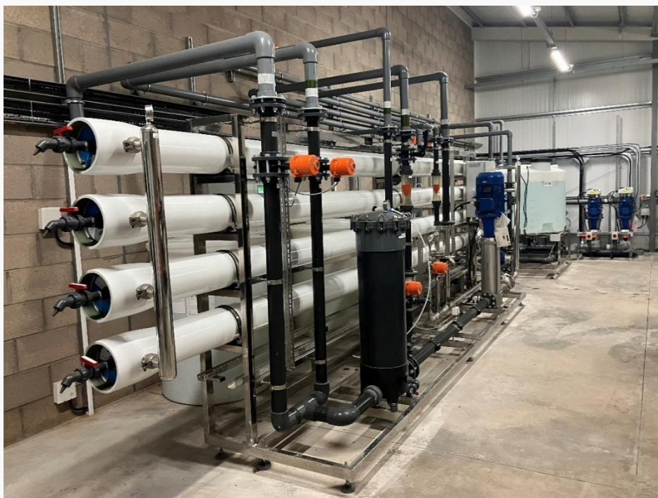
Figure 12 A membrane filtration system at a large regulated private water supply.
