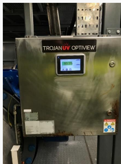
Figure 4 A UV monitor at a WTW in the North East of Scotland
