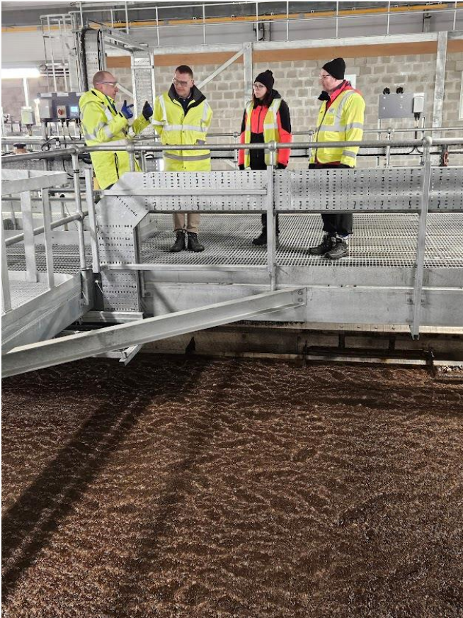
Figure 10 DWQR observing a filter back wash at a WTW in Northeast Scotland.
