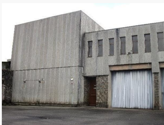
Figure 1 A large WTW in the west of Scotland.
