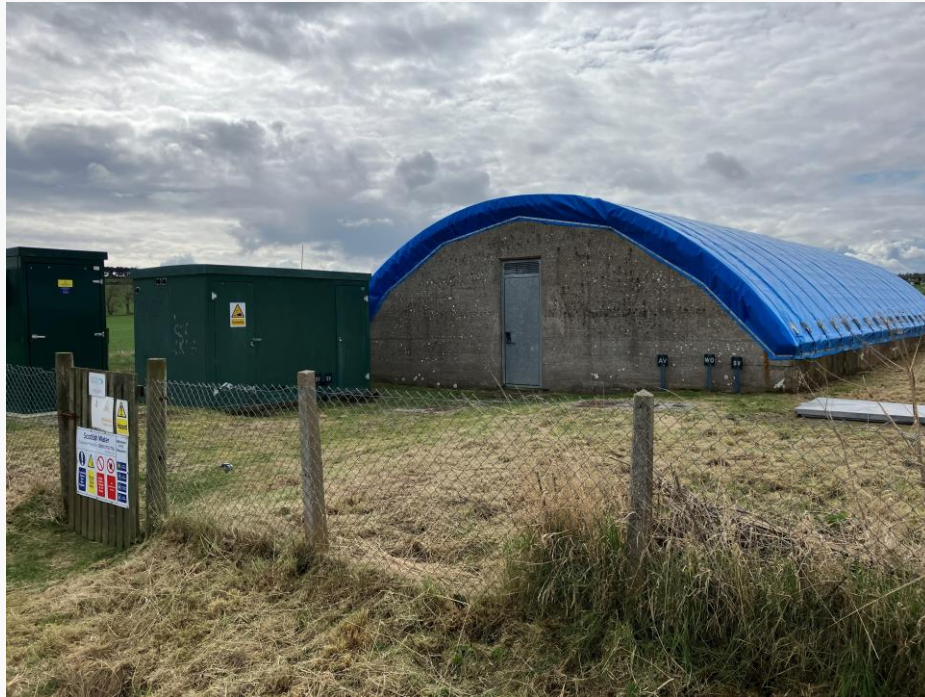
Figure 14 An example of temporary mitigation at an SR in the North of Scotland.
