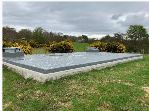
Figure 16 SR after repair
