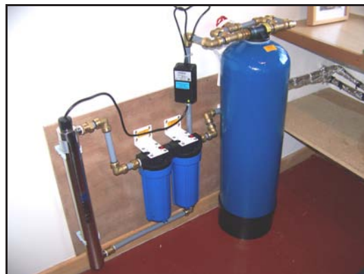
Water treatment at a PWS
