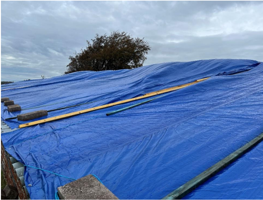
Image 5 Temporary Protection at Darvel SR (Since Fully Repaired and Restored to Service)
