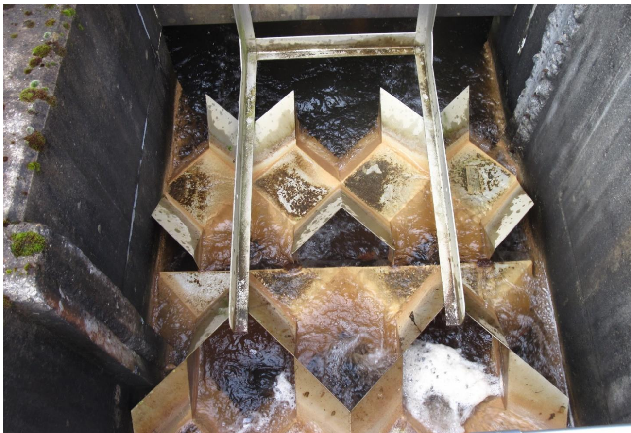
Image 8 Coagulation Chemical Mixing at Water Treatment Works
