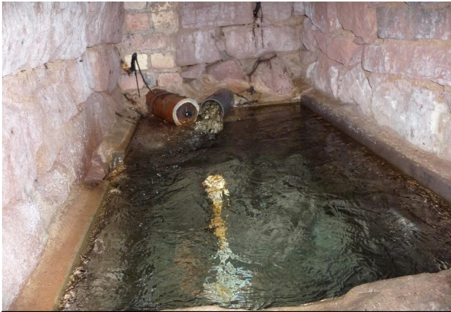
An underground Private Water Supply source in the South of Scotland
