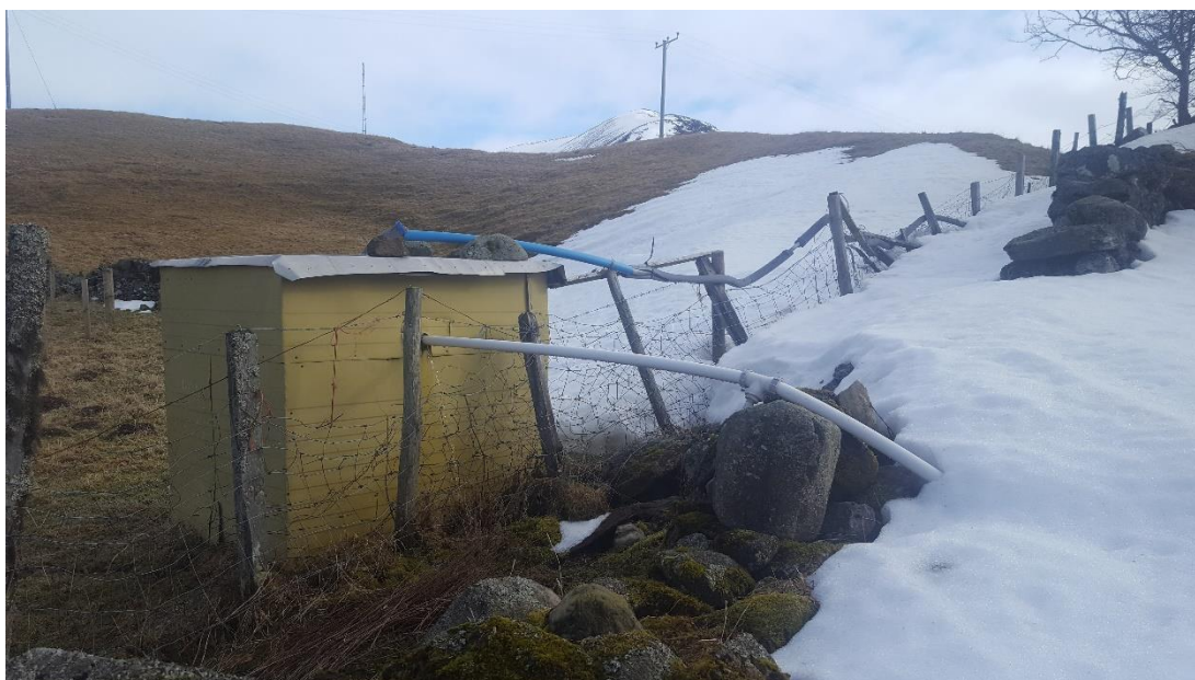
A Private Water Supply Storage Tank in the Cairngorms with Dubious Construction
