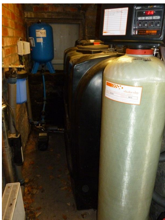
Example of a fibreglass shell particulate filter (pale vessel), with on-site storage of treated water (black tank)
