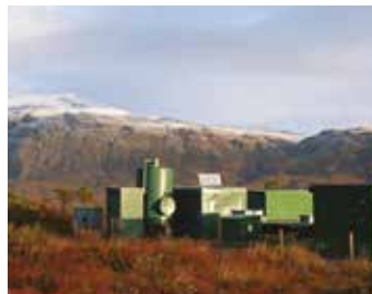
252 Water Treatment Works
