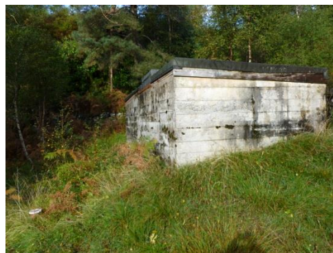
PWS collecting tank
