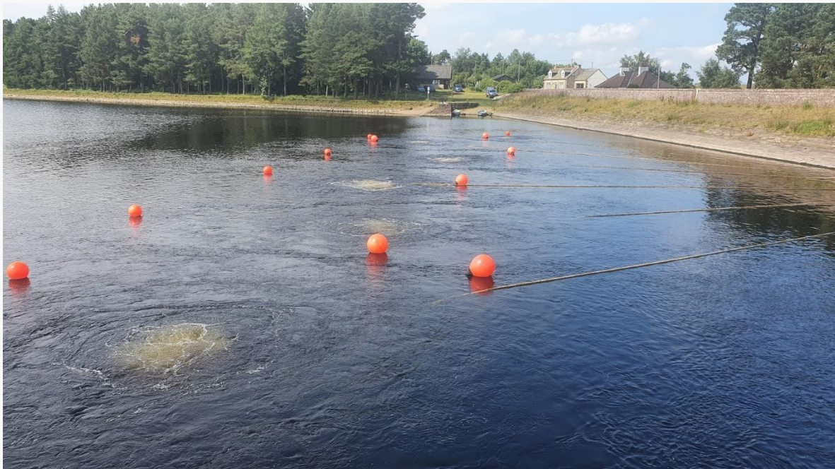
Figure 8 Bubble curtain used to disrupt algal growth.
