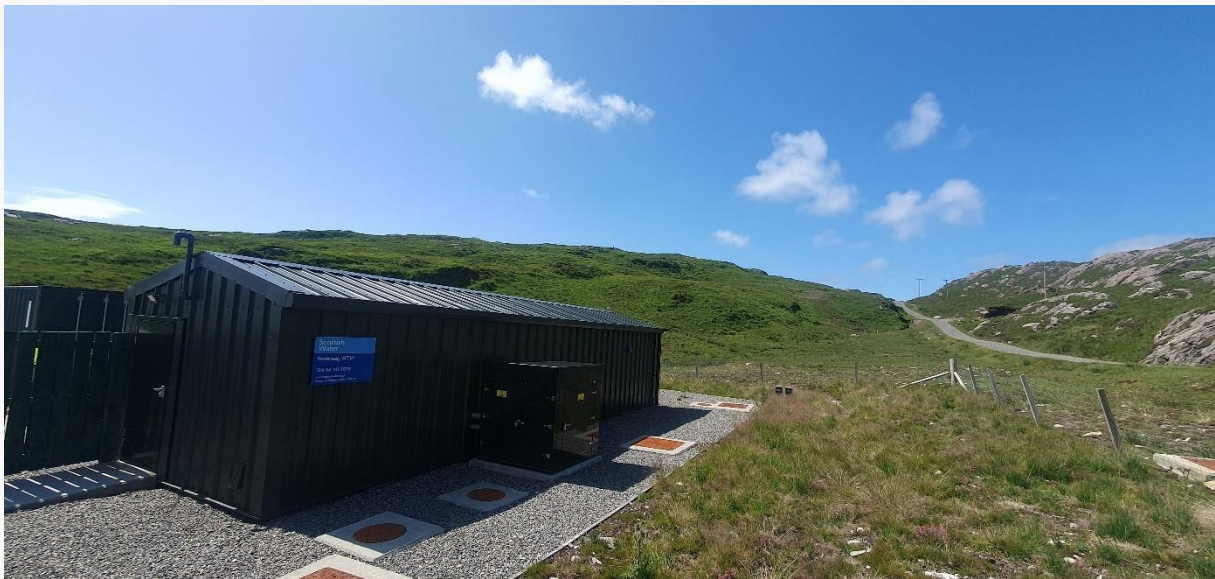
Figure 1 A small water treatment works in the Western Isles.
