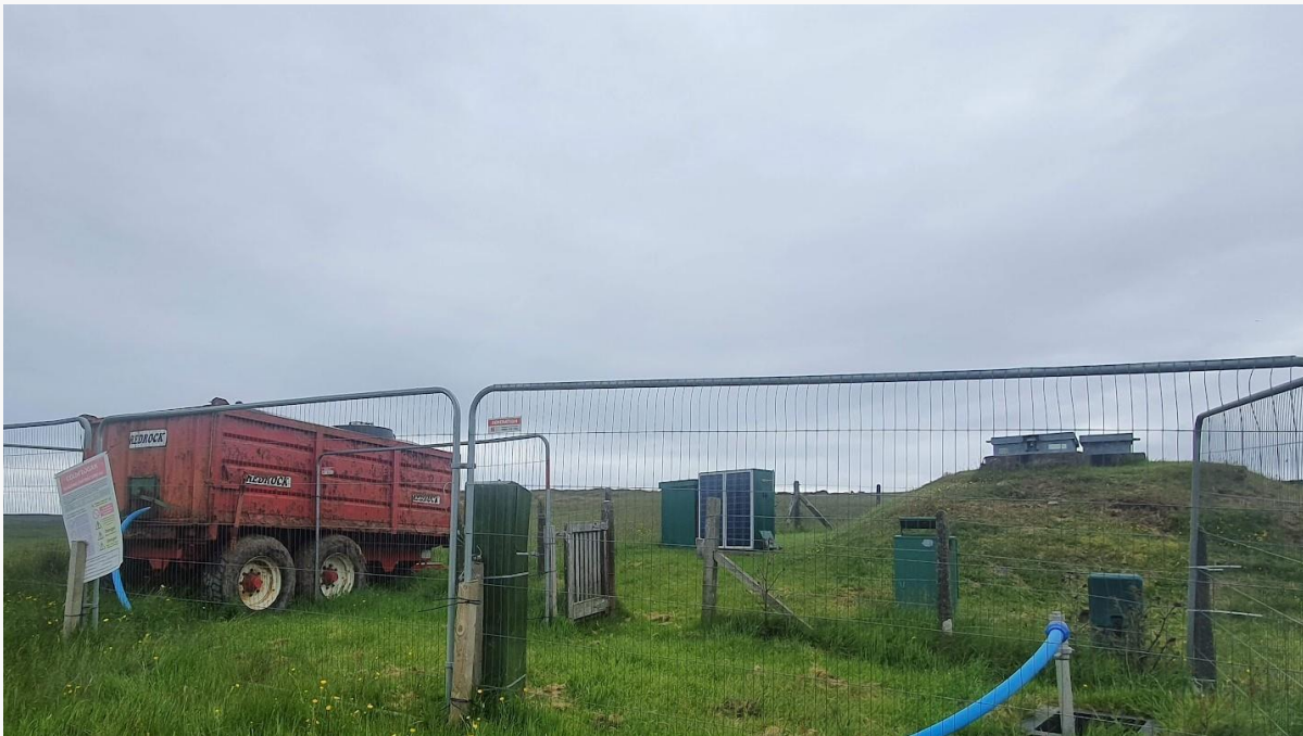
Figure 3 A temporary tank that was audited by DWQR.
