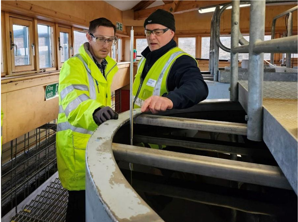
Figure 16 Top: WTW CWT Bottom: A demonstration of a Dynasand filter
