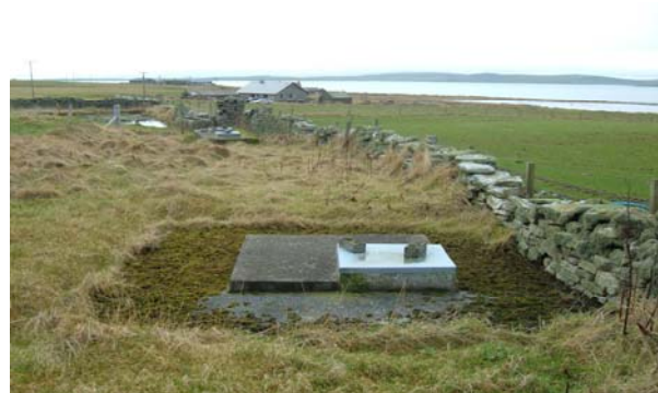
Part of Papa Westray Community Supply, the first supply in Scotland to develop a Water Safety Plan (WSP).
